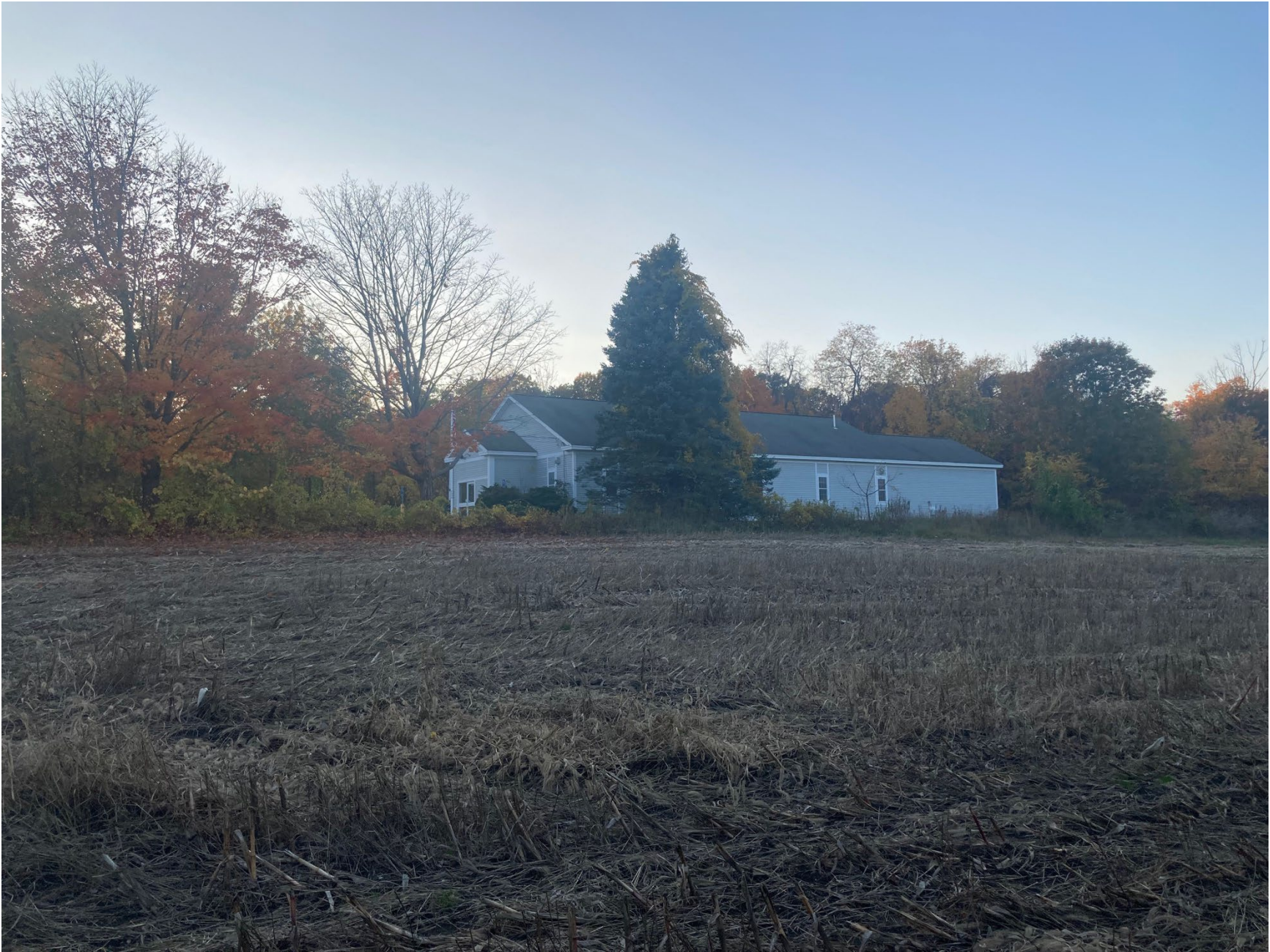
Photo 4 North West View of Post Office from Access Road Entrance
