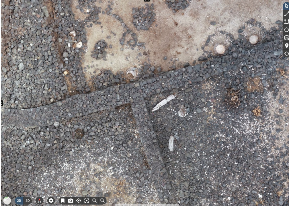
Figure 5-4. Walls visualized from low level drone flights using photogrammetry.
