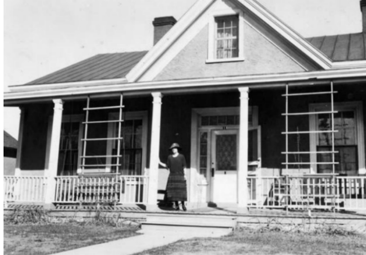
Figure 4-7. Photo from 1920 of R.N. Miller House at 123 Grant Avenue, whose location is within the project area. (Image from Montoya 2023)
